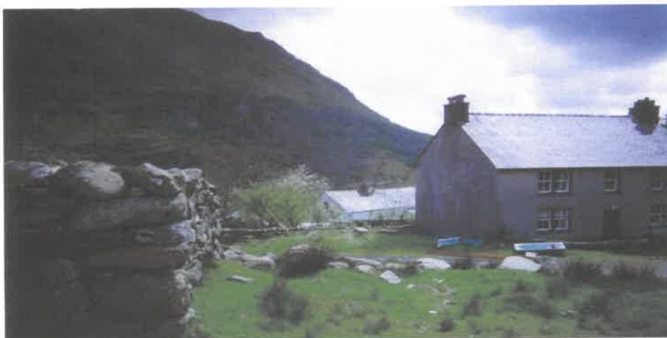
Fig 6, The new house.
