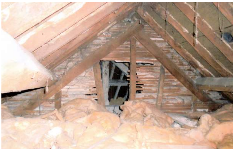
The attic space showing the lath and plaster partition.
