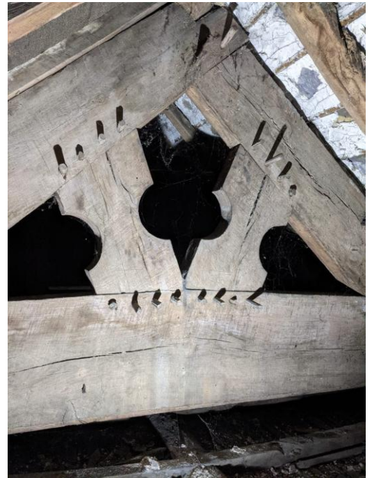
Brynmor carved attic beams (photograph: Eleanor Carpenter)
