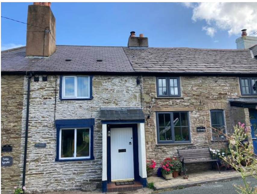
Bradford House (left) and neighbouring house with graded slates
