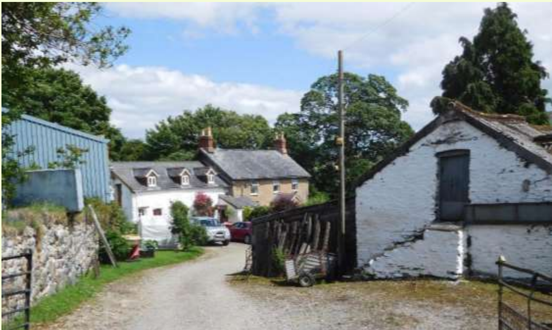
Tyn y Celyn with older house part to the left and 'newer' house to the right (Jenny Lees)
